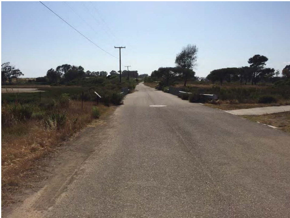
Photo: 8-Looking from east to west along Venoco Crossing.
