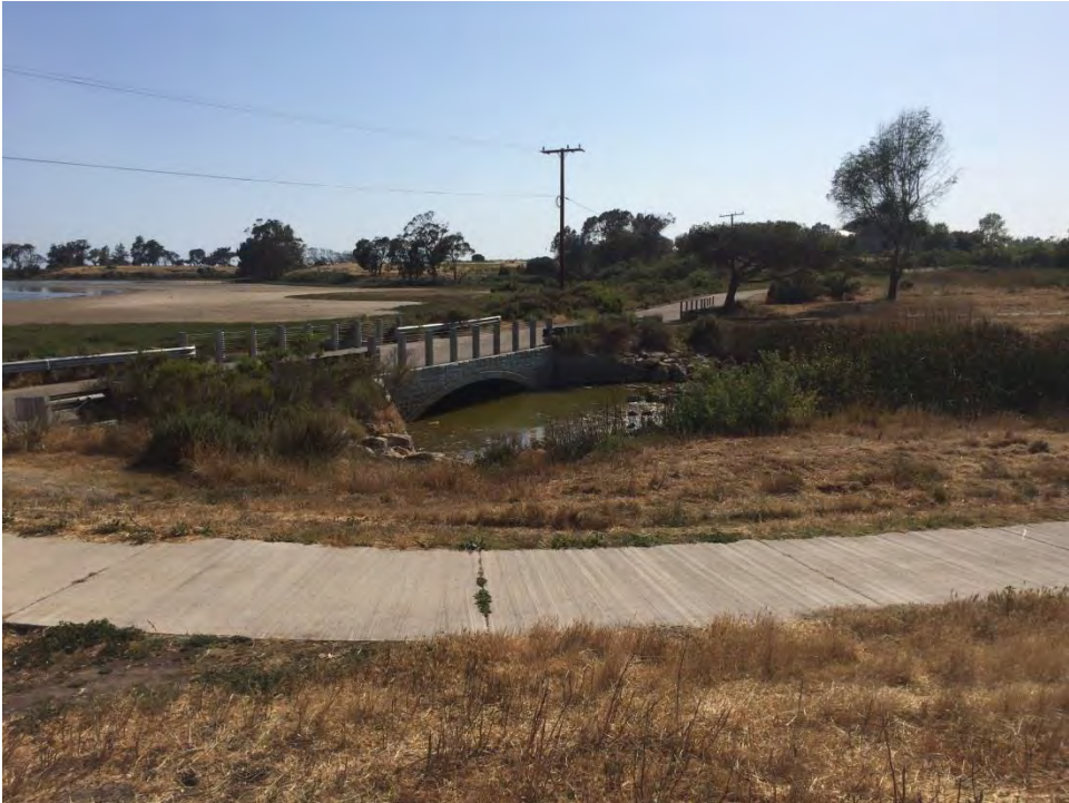
Photo: 10-Upstream side of Venoco Crossing
