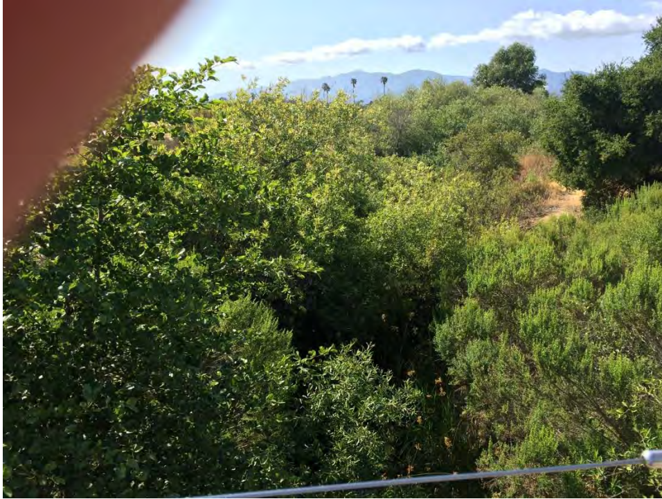
Photo: 1 - Looking upstream from Marymount Way. Vegetation forms an open tunnel that shades the bottom and prevents for better flow characteristics.
