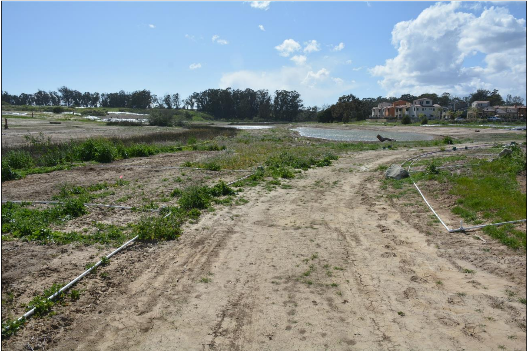
As-built photo - April 16, 2018.
