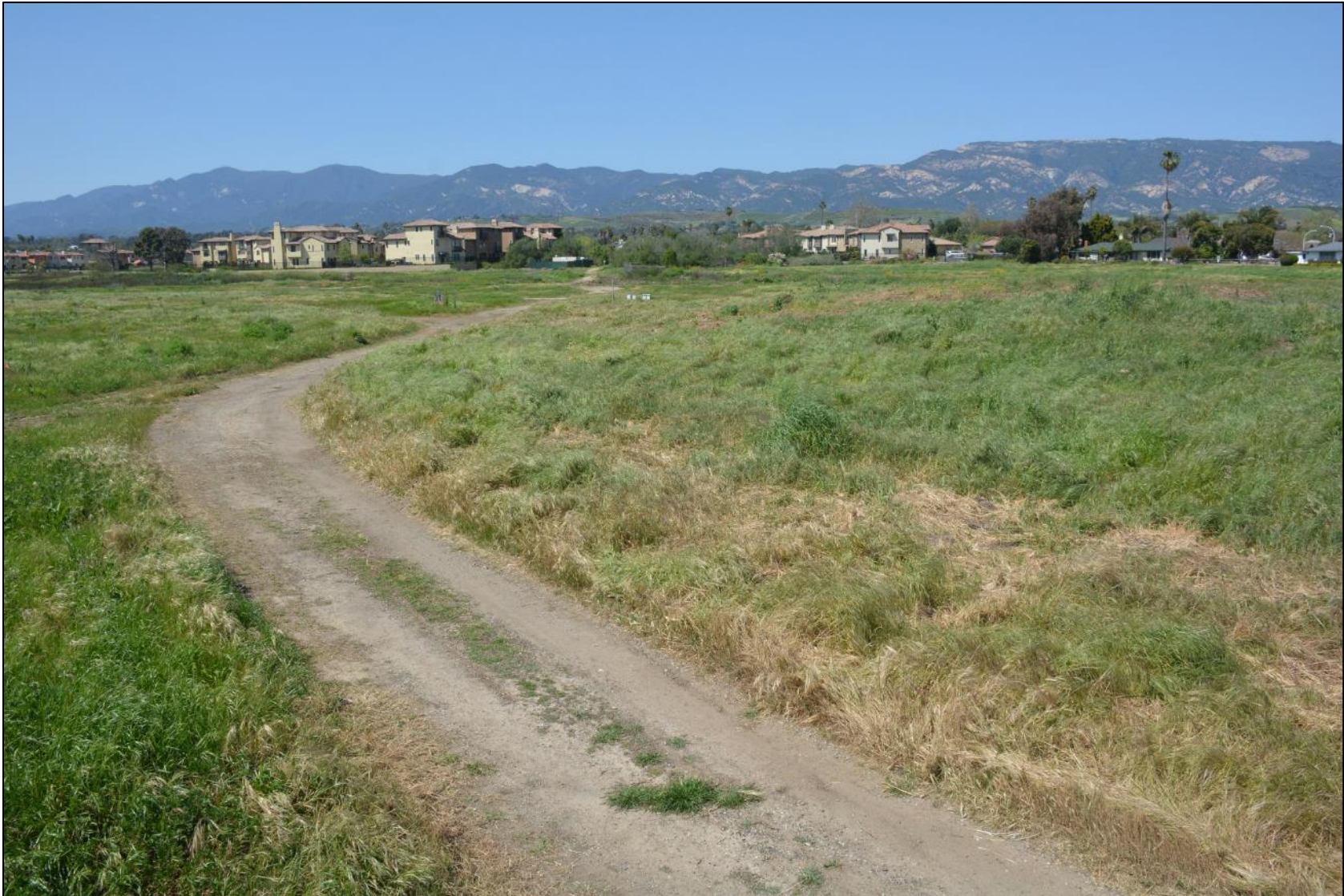
Baseline photo – pre-grading, April 10, 2017.
