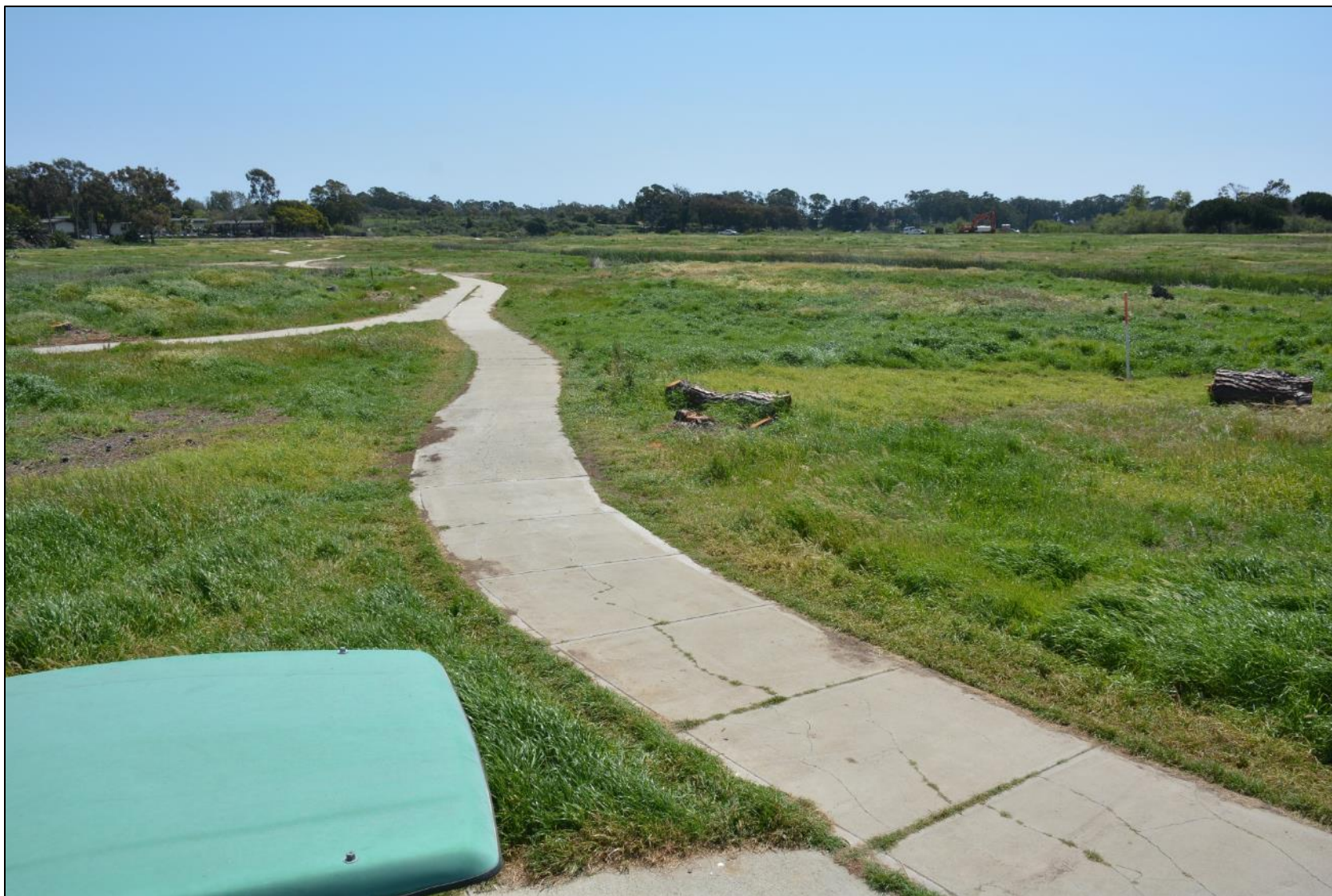
Baseline photo – pre-grading, April 10, 2017.
