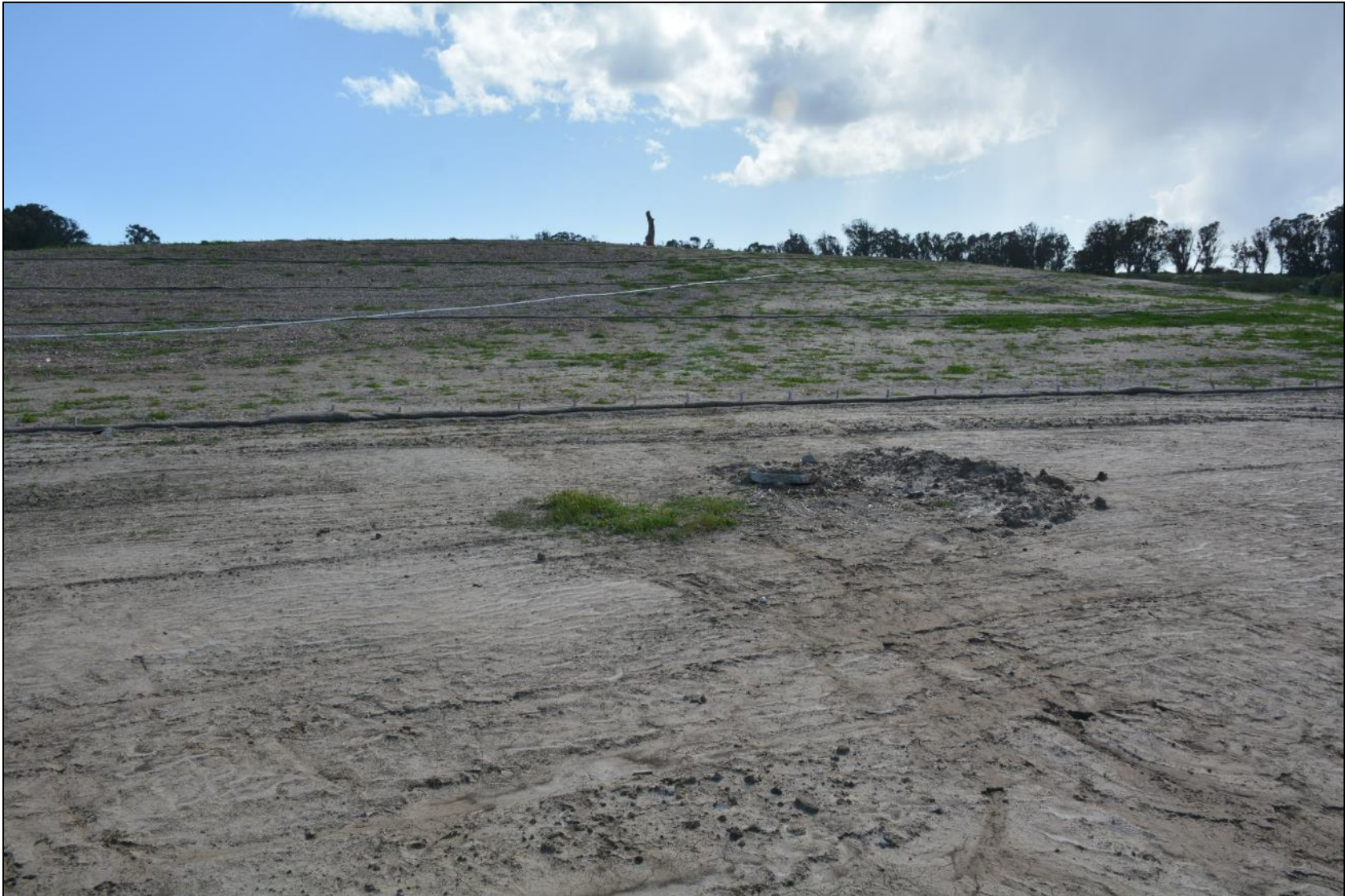
As-built photo - April 16, 2018.
