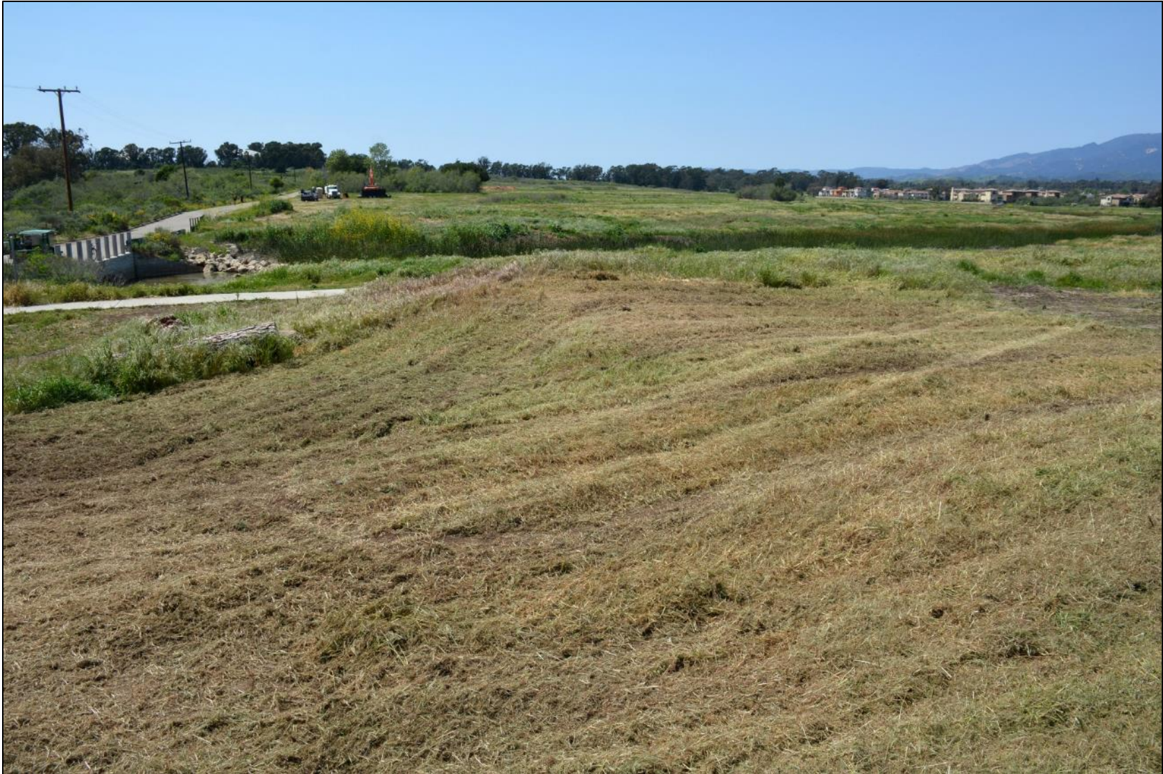
Baseline photo – pre-grading, April 10, 2017.
