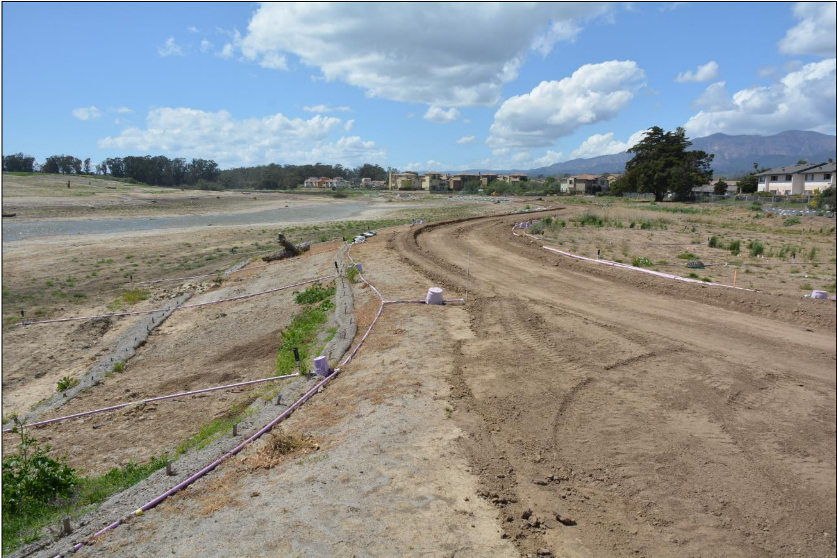
As-built photo - April 16, 2018.
