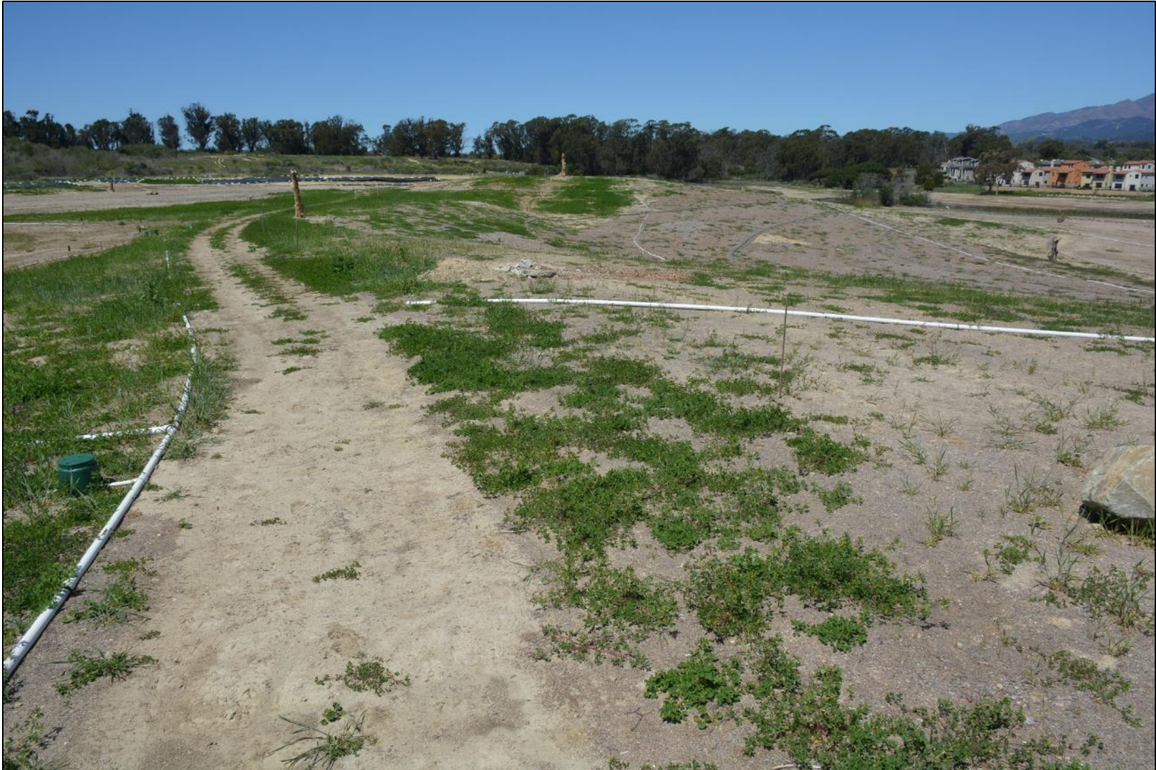
As-built photo - April 17, 2018.
