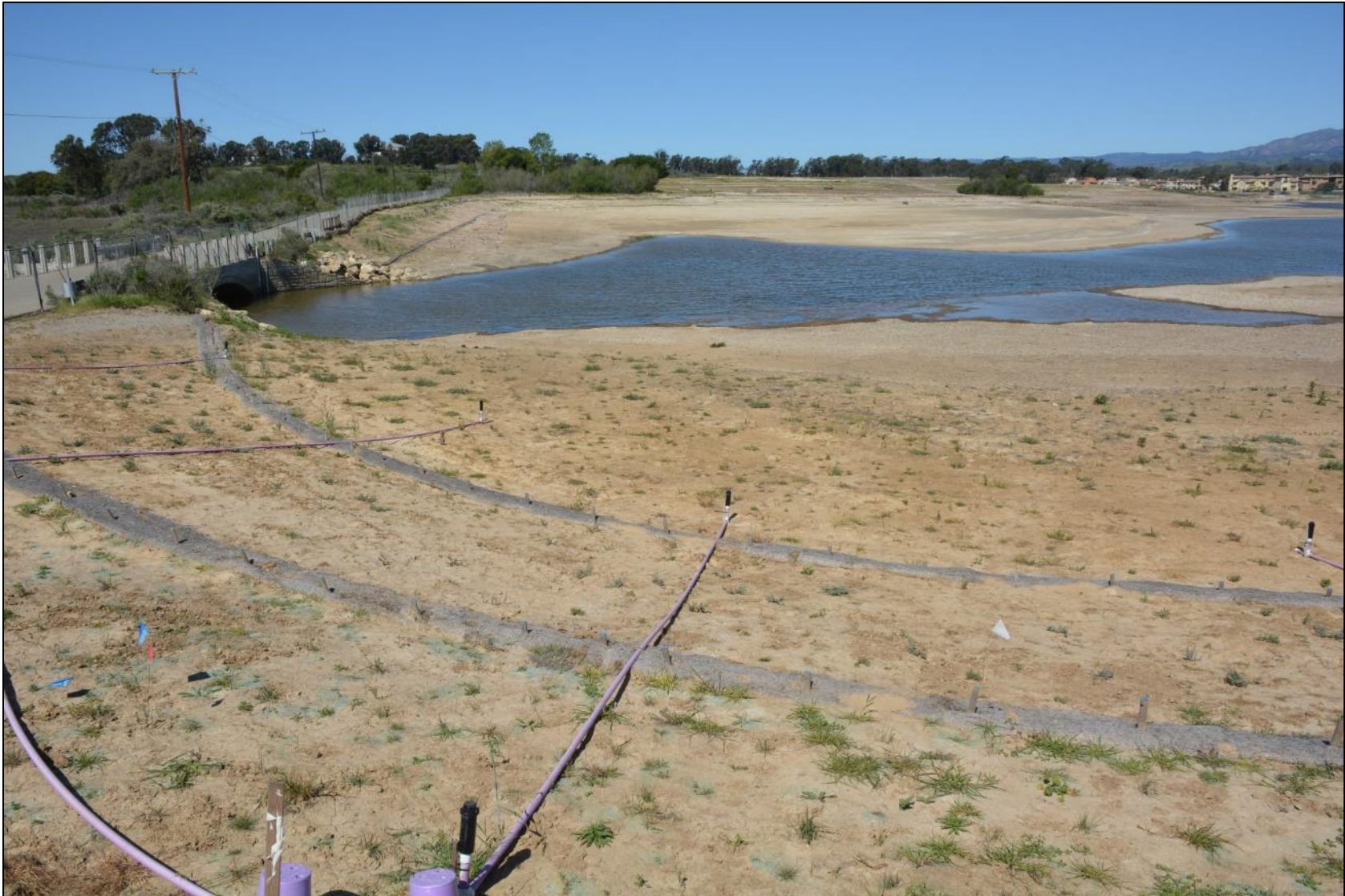
As-built photo - April 17, 2018.
