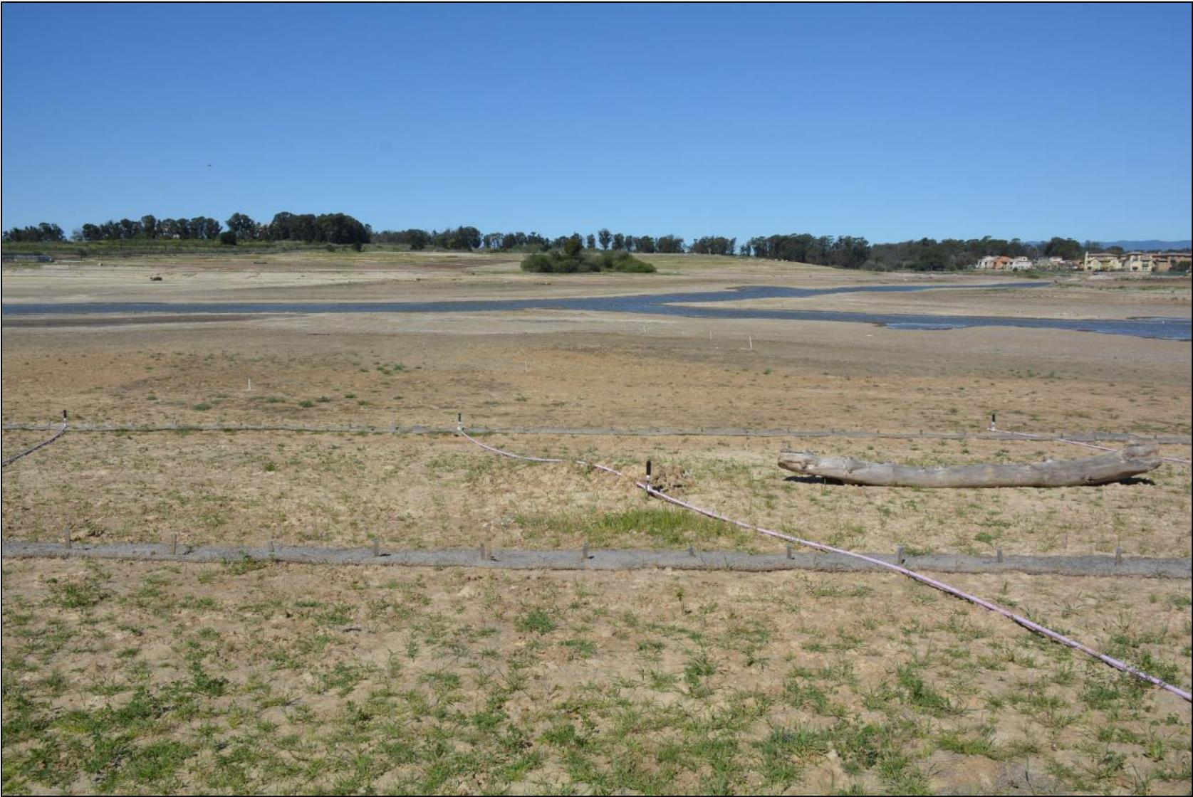
As-built photo - April 17, 2018.
